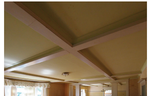
Living Room ceiling
