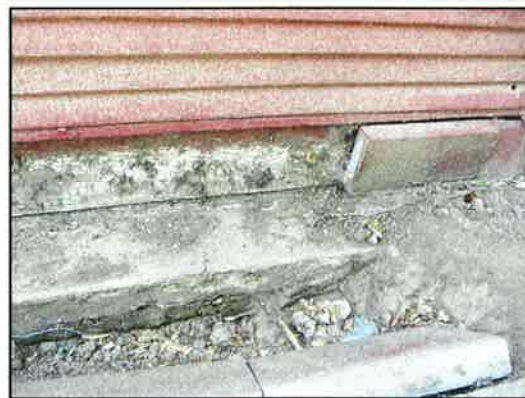
Soil at Sill Plate Level
