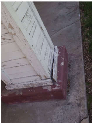
Porch Column base
