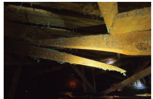
Broken joist
