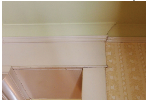
Living Room molding and ceiling
