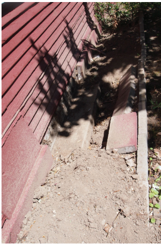
Bottom of wall at grade
