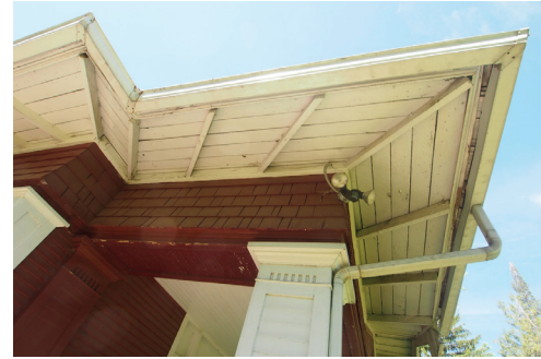
Radial joists at front porch
