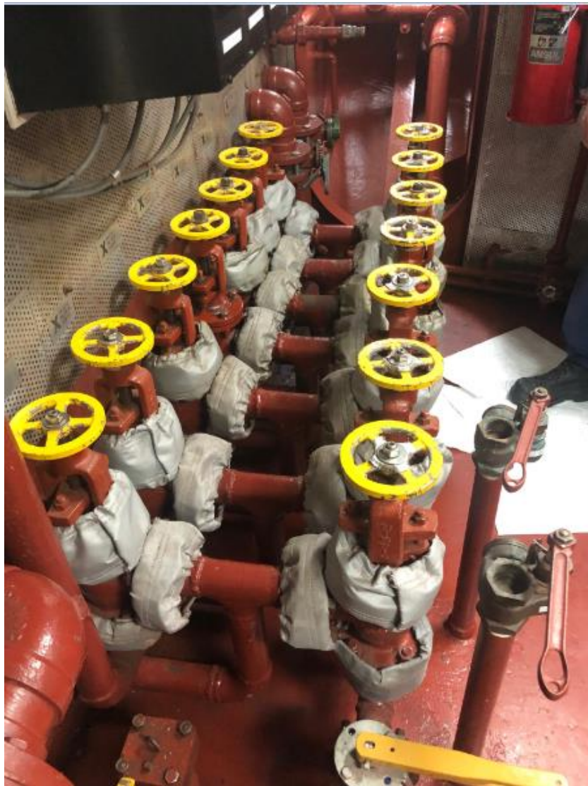
FIGURE 1. PHOTO OF FUEL MANIFOLD ASSEMBLY
