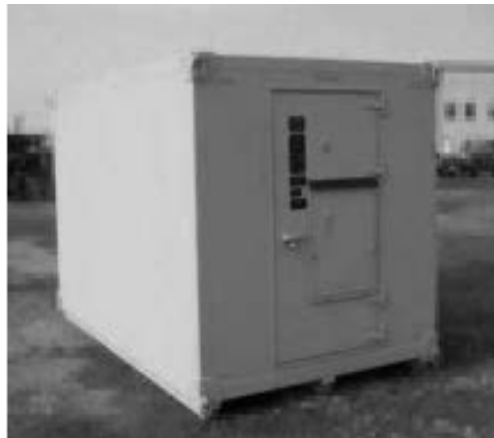
Figure 1. Personnel Door and Emergency Exit Panel: Outside View.
