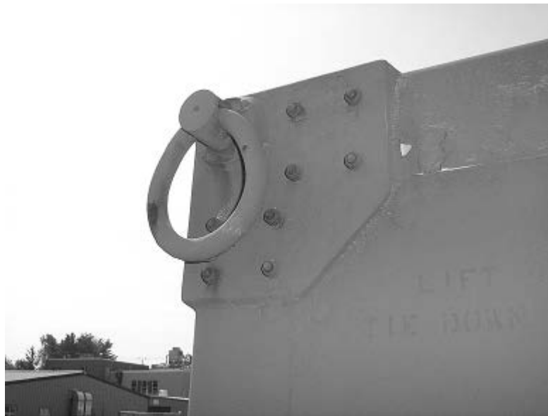
Figure 1. Lifting and Tiedown Eye Assembly.
