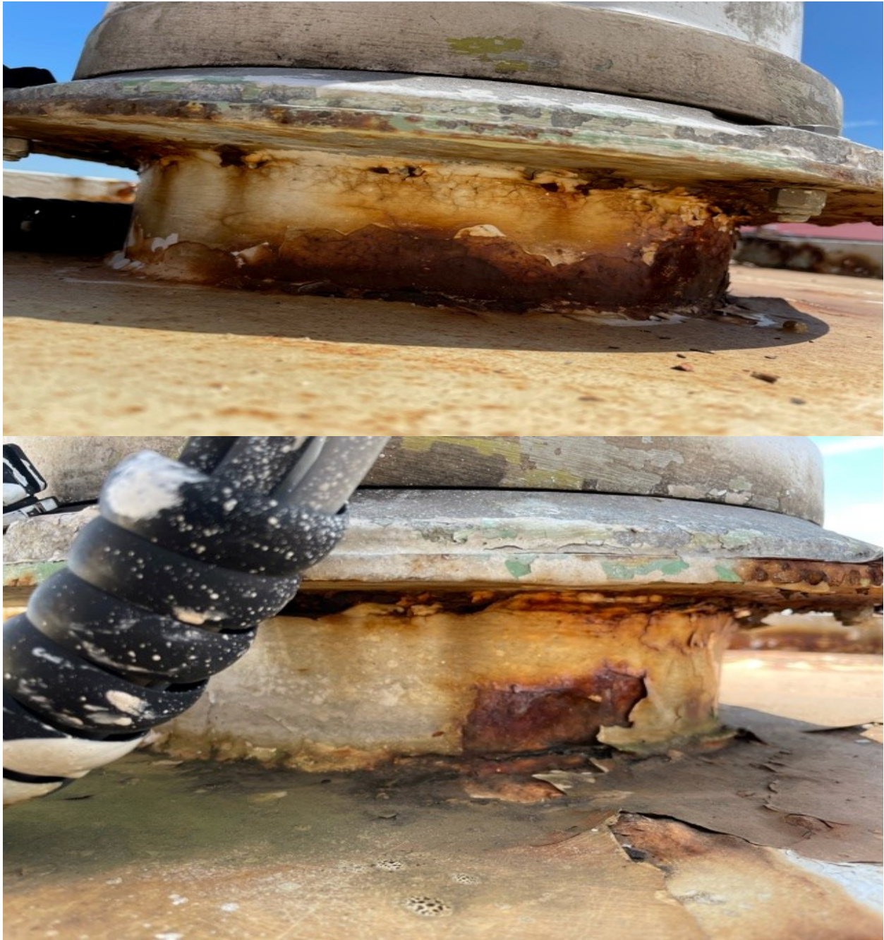
PHOTO 1: PORT AND STBD SEARCHLIGHT FOUNDATIONS
