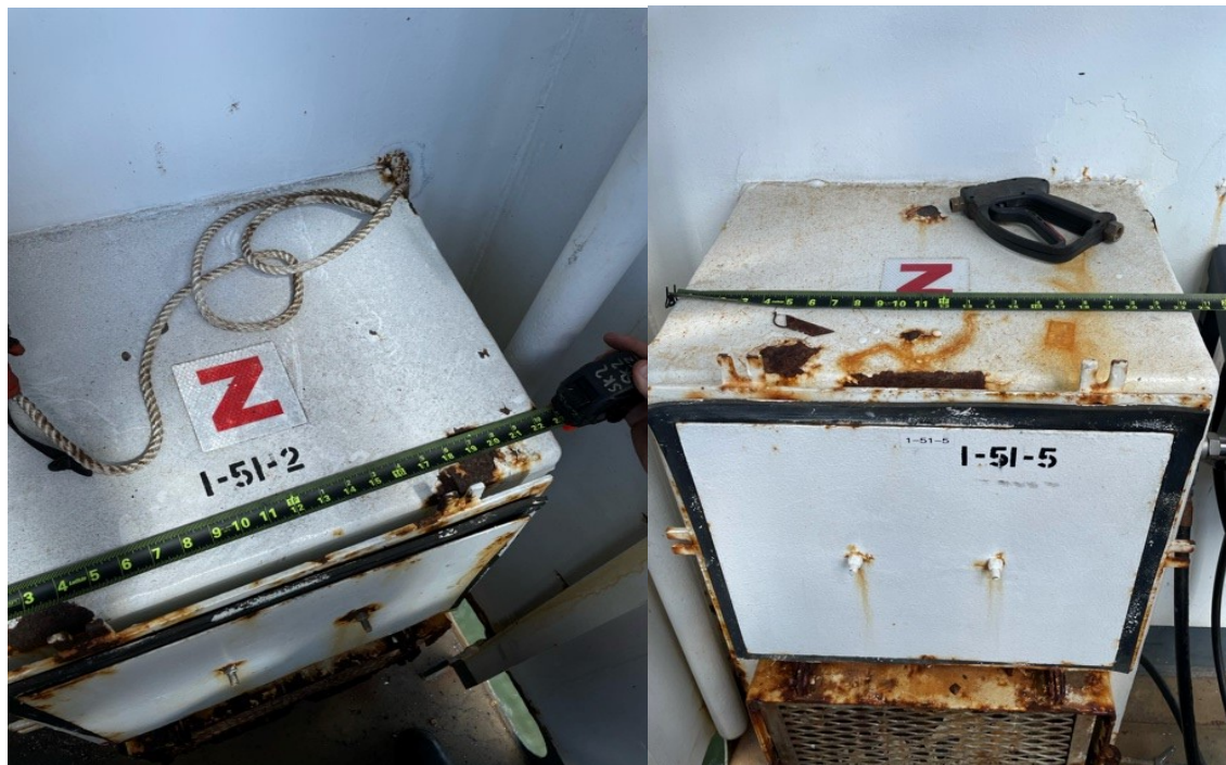
PHOTO 1: BUOY-DECK VENT DUCTS
