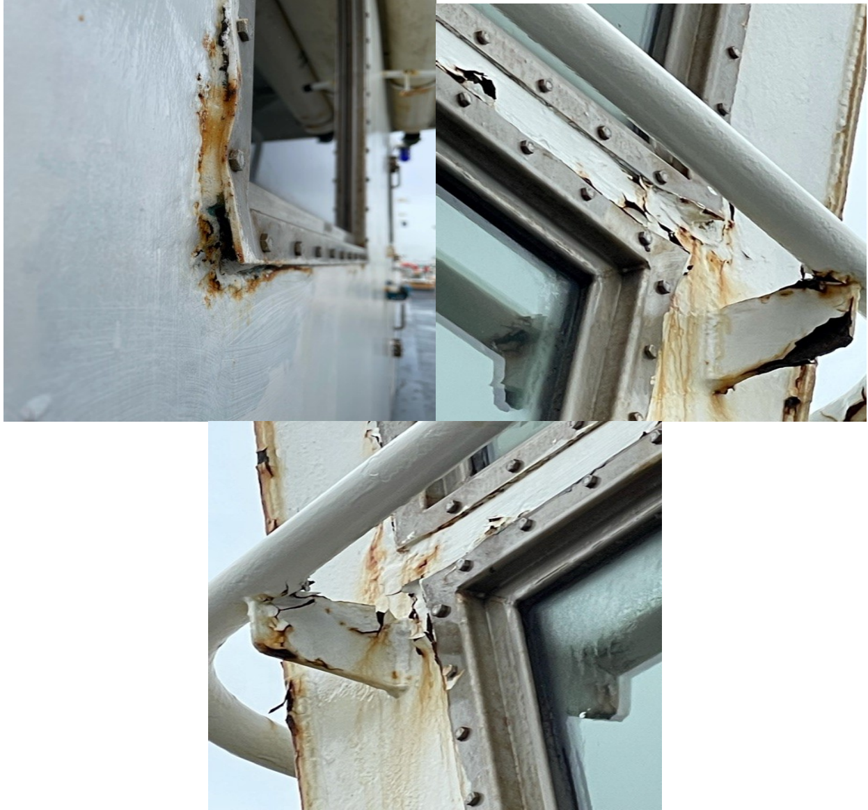
PHOTO 1: PILOT HOUSE WINDOWS
