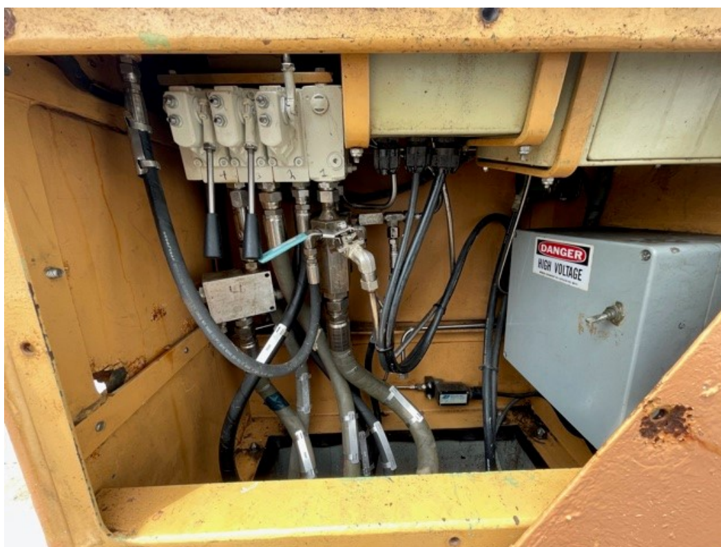
PHOTO 2: SMALL BOAT DAVIT CONSOLE FOUNDATION, INTERFERENCES
