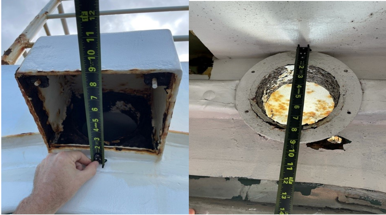
PHOTO 3: STORAGE LOCKER FANTAIL VENT
