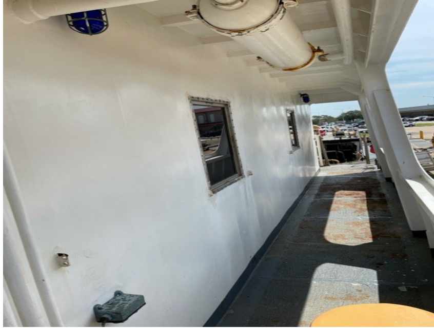
PHOTO 2: WINDOWS ON THE 01-DECK
