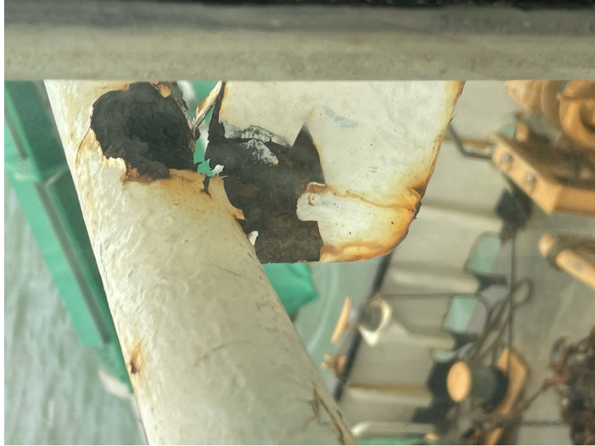
PHOTO 2: HANDRAILS MOUNTS JOINTS
