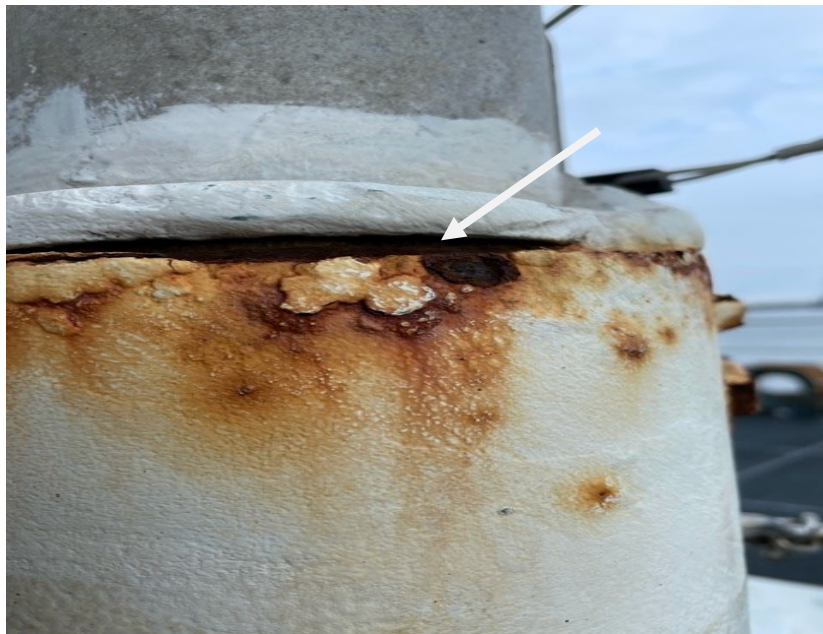
PHOTO 2: LINER SLEEVE RENEW
