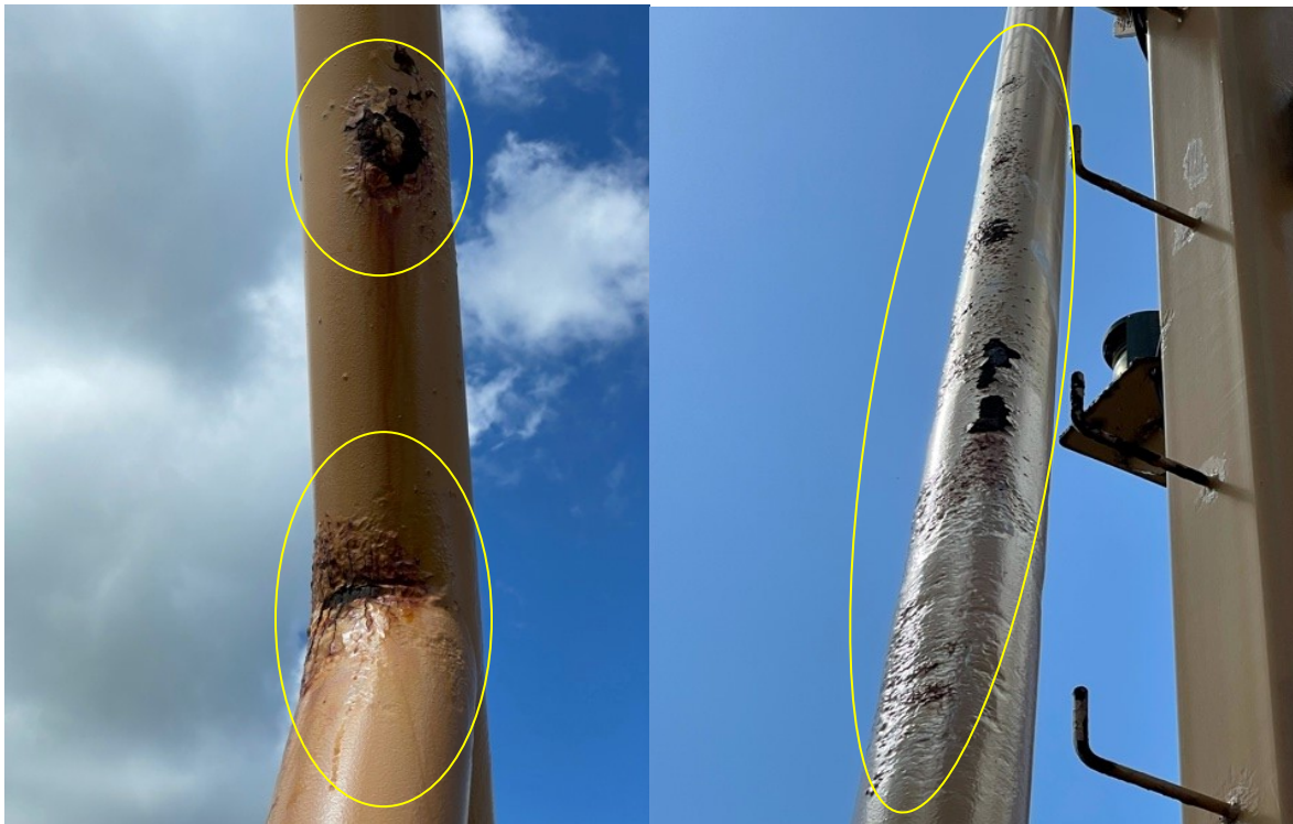
PHOTO1: FWD MAST SUPPORT PIPE
