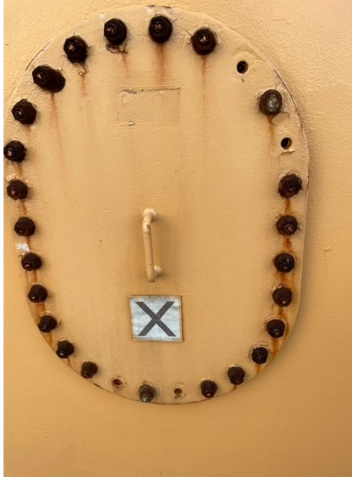
PHOTO 1: EXHAUST STACK INSPECTION COVER
