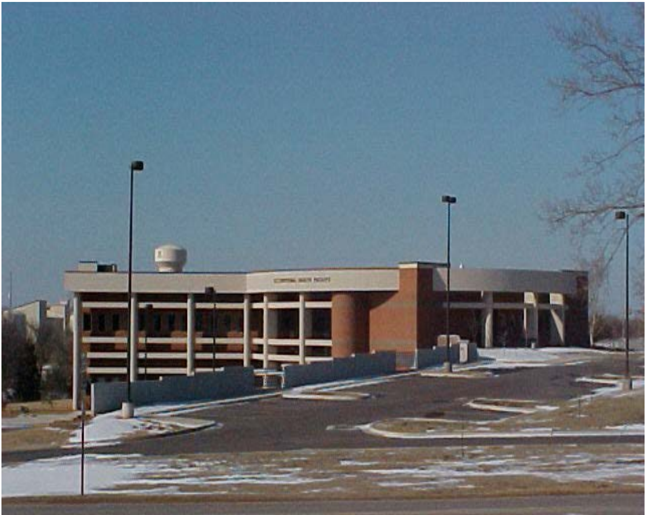
Occupational Health Facility TAFB
