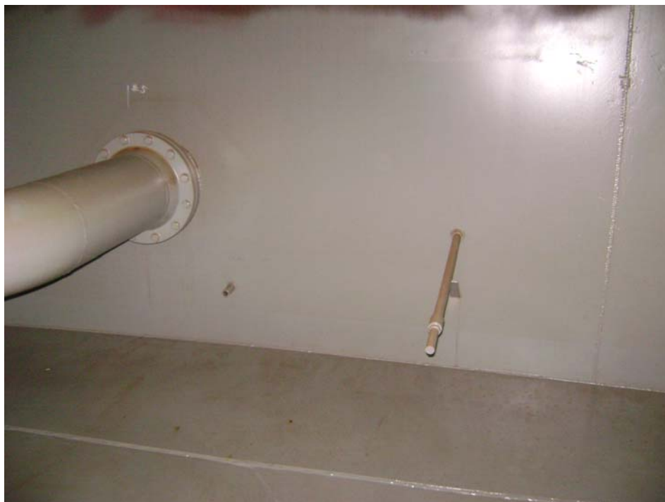
Left to Right: 12" Fill Nozzle, 1" Thermal Relief Nozzle and Temperature Thermowell (Not Used)
