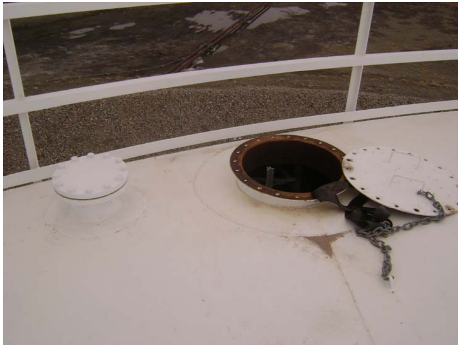
10" Nozzle with Blind and 24" Diameter Roof Manway
