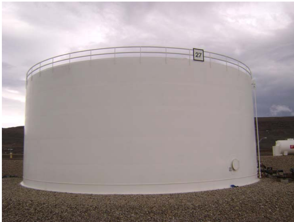
Tank 27 – West Elevation
