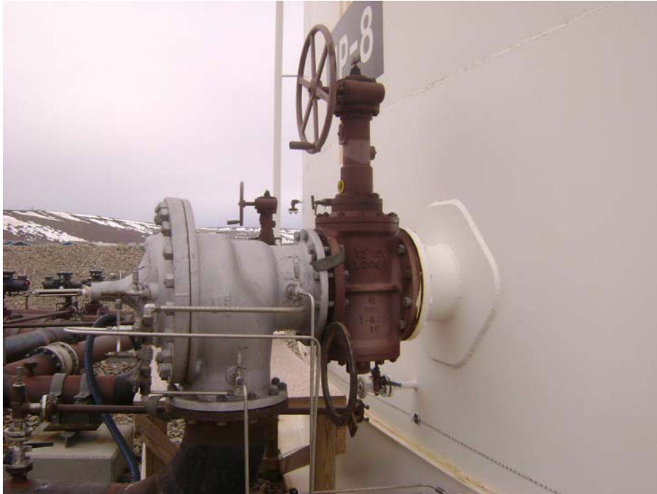
12" Fill Nozzle with HLV Pilot Tubing and 1" Pressure Relief
