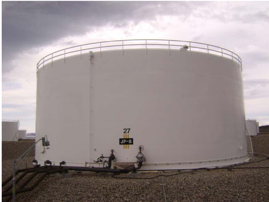
Tank 27 – South Elevation
