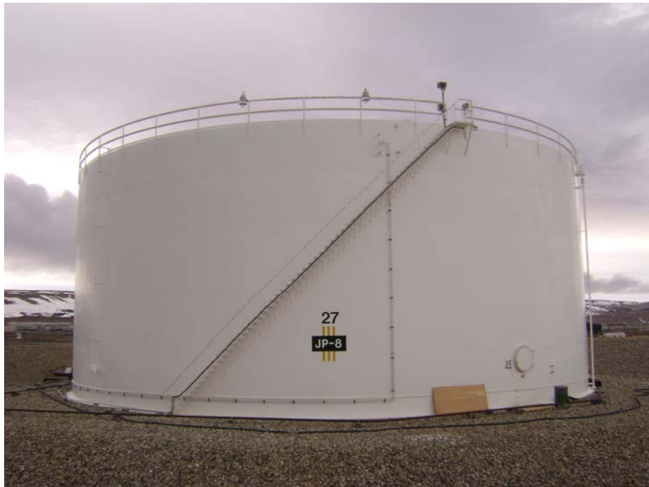
Tank 27 – East Elevation
