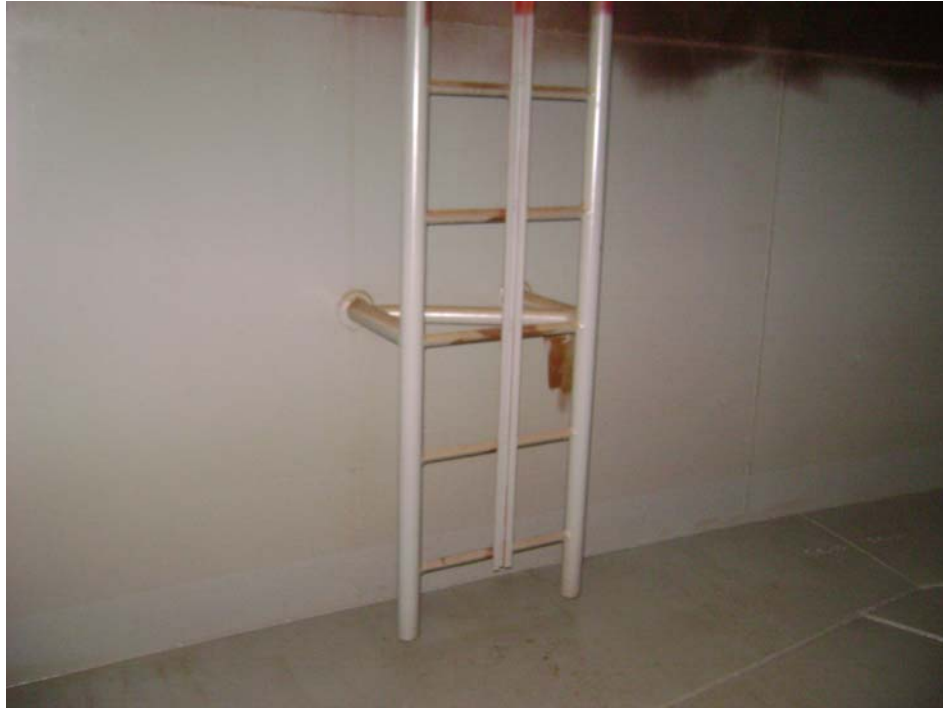
Roof Access Ladder
