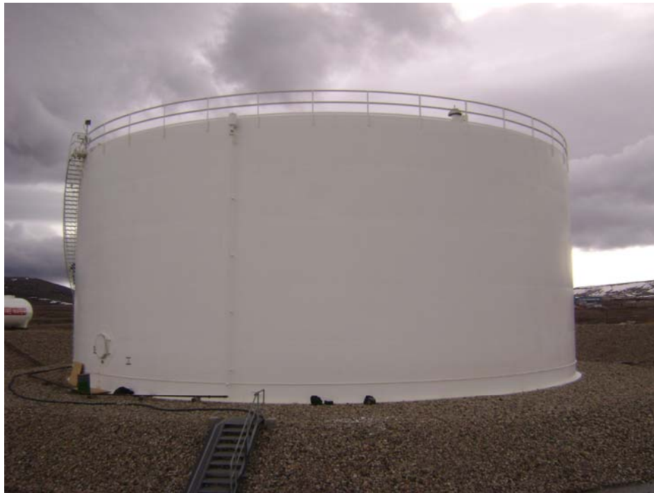
Tank 27 – North Elevation
