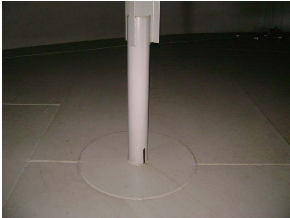
Roof Support Column (Typical of 16)
