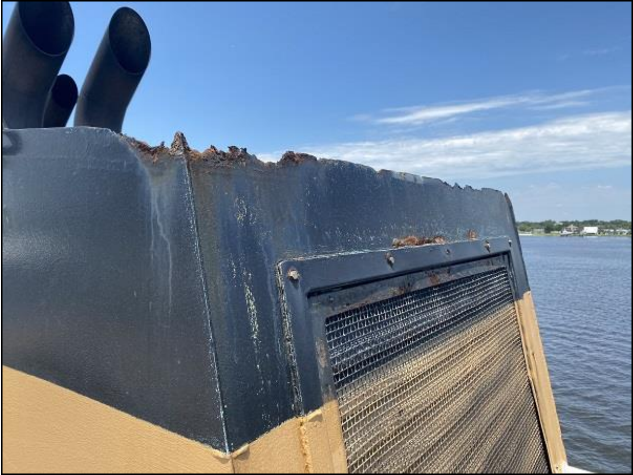
PHOTO 2. EXHAUST STACK WORK AREA
