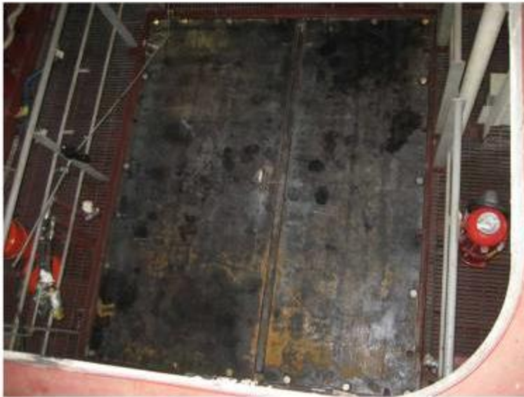
Figure, Z-drive Sea Well Covers Installed
