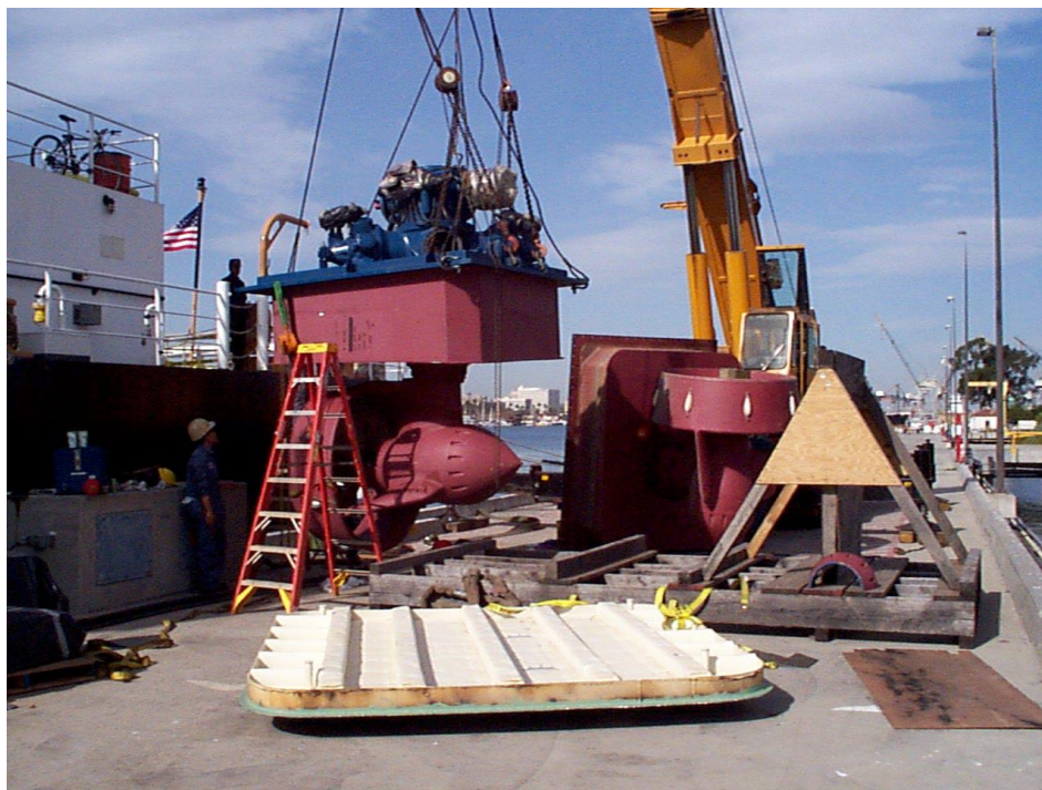
FIGURE 2. HISTORIC Z-DRIVE LIFTING ON-OFF CUTTER PHOTOGRAPH
