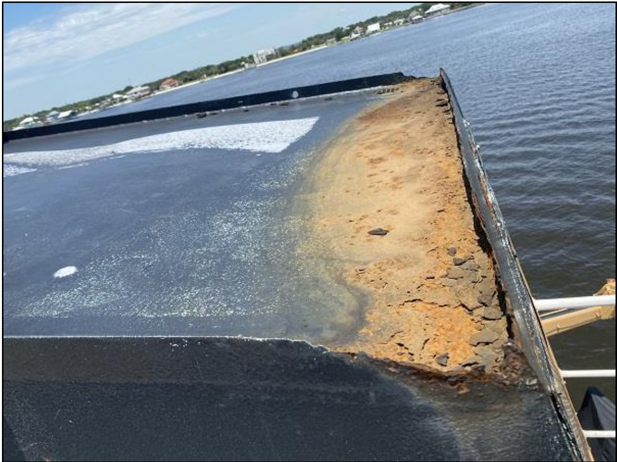
PHOTO 1. EXHAUST STACK WORK AREA
