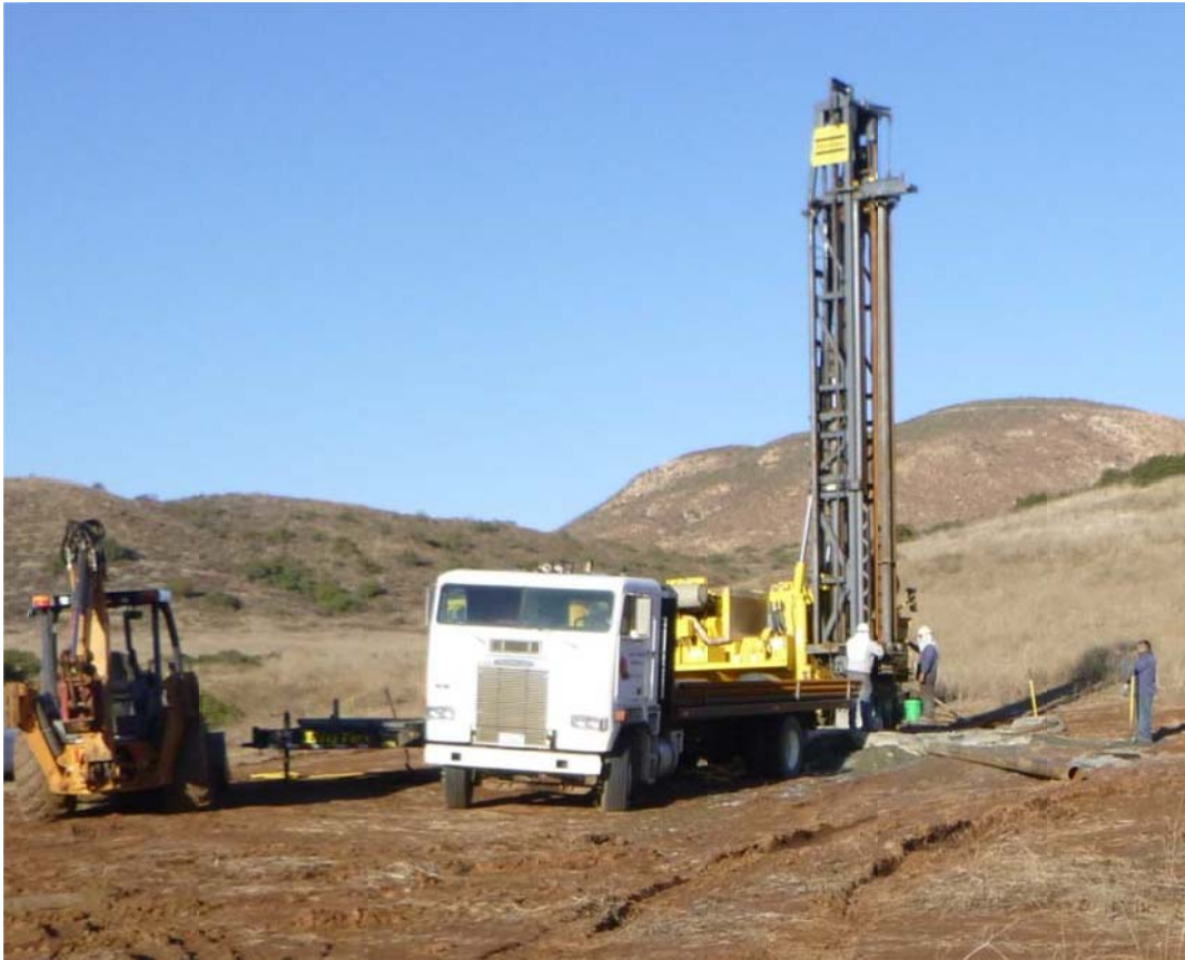
Figure 2-3 Installation of 8 5 / 8 -inch Casing
