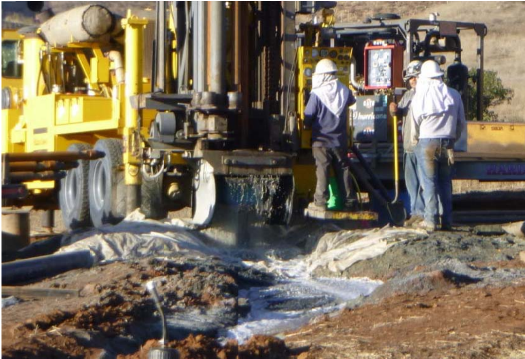
Figure 2-2 Mud Rotary Drill Rig
