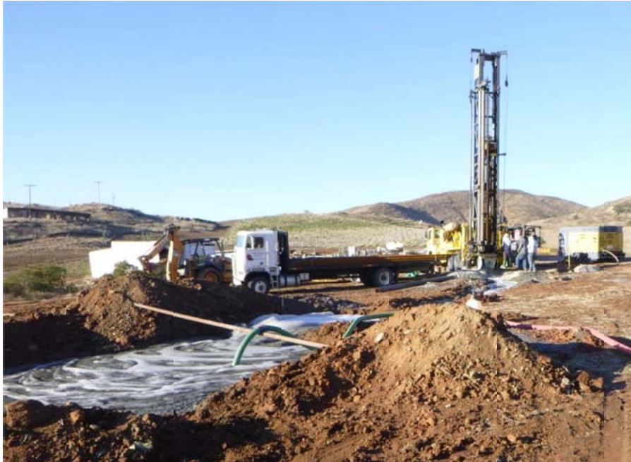
Figure 2-5 Water Discharge during Well Development
