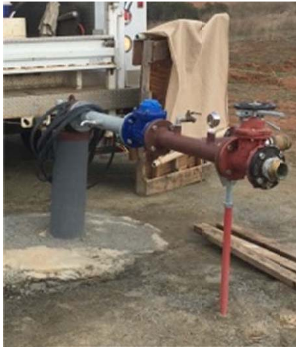
Figure 3-1 Pump Valve for Water Quality Sample Collection
