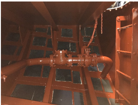
Inside Void 3-78-2, looking outboard
