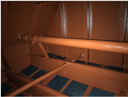
Pipe penetration inboard bulkhead of Void 3-78-2
