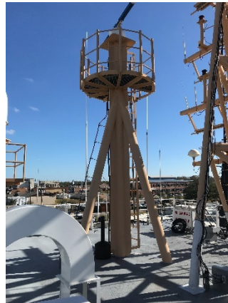
X-Band Radar Mast
