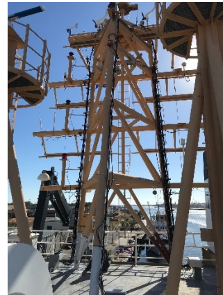
Main Mast (looking aft)
