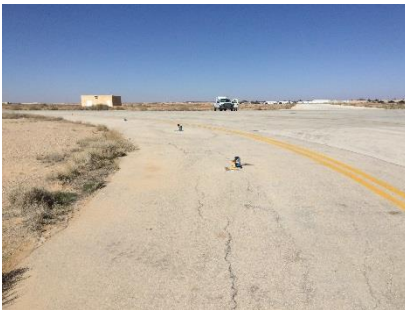
Taxiways Lima 4 / Lima Intersection. Taxiway Lima 5, Straight Ahead.
