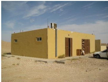
Vault B: Exterior view.
