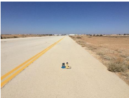
Taxiway Lima 5, Temporary Solar taxiway Edge Light supplementing permanent light fixture.
