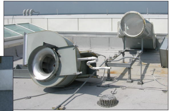
Figure 8. The equipment on this stand was resting on vibration isolators that provided lateral resistance but no uplift resistance (above). A damaged vibration isolator is shown in the inset (left).
