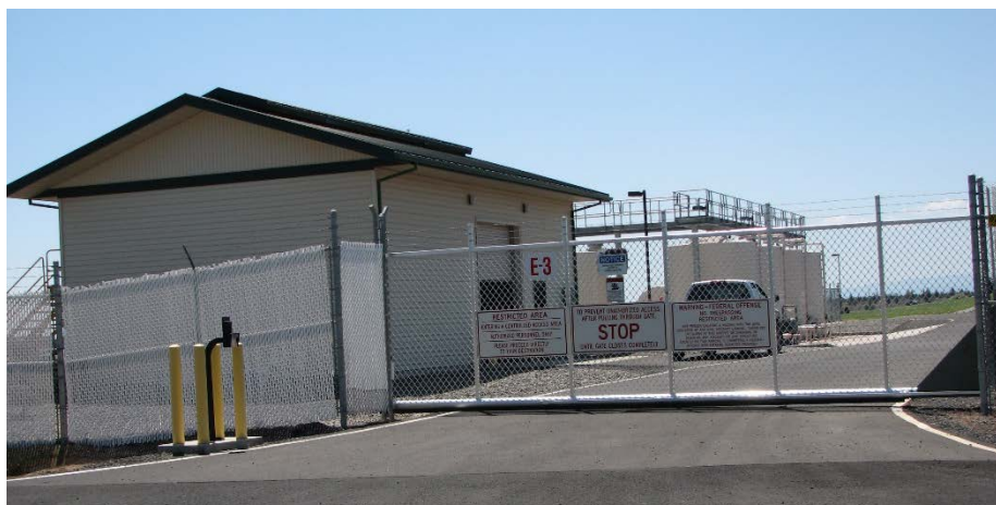
Electronic Gate Using Proximity Card Access Control
