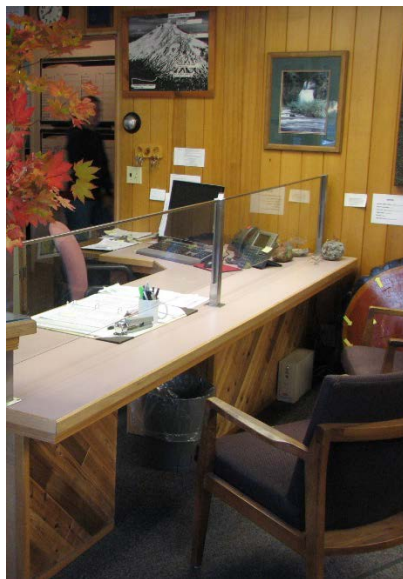
Protective Glass at Accessible Counter
