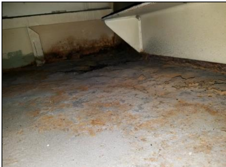
PHOTO 3, 03 DECK IN STACK
