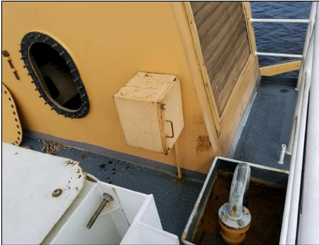
PHOTO 1, WORK LOCATION STACK AND COAMING
