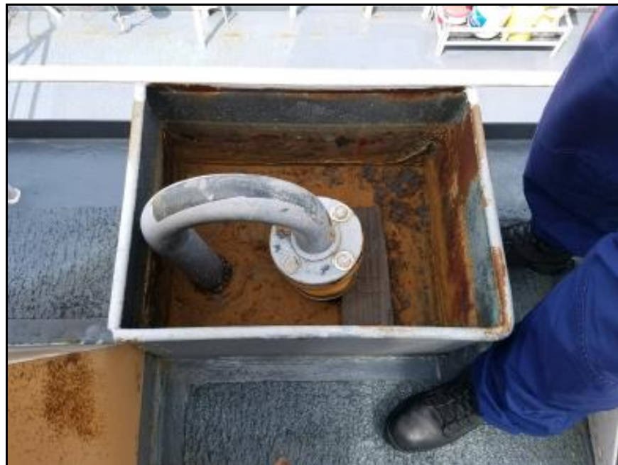
PHOTO 2, COAMING, FUEL SERVICE TANK (02-77-1-F)
