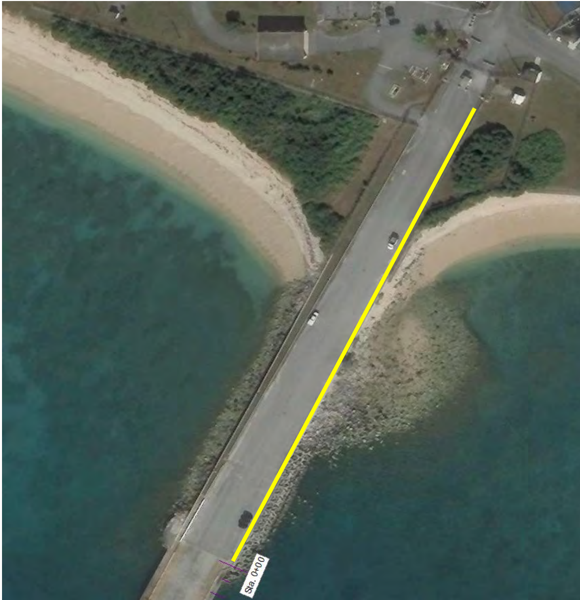
Figure 6-1. Aerial View of Shore Attached Causeway
