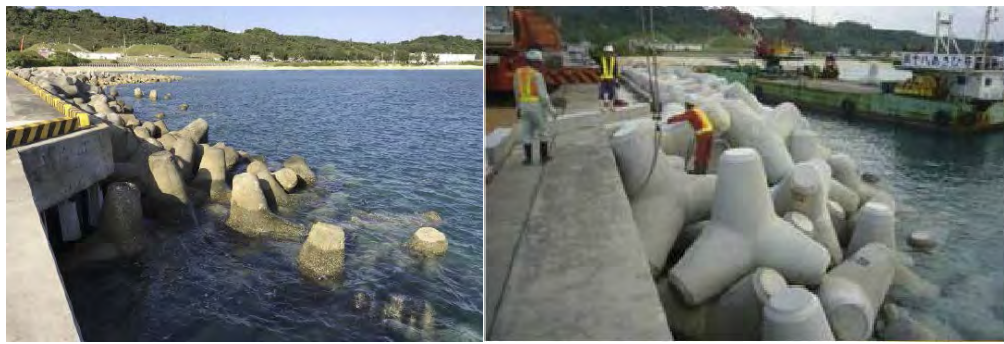
Insert 6-1. Tetrapods at White Beach Fuel Pier, 3 Nov 2007 (L) and 2 April 2018 (R)
