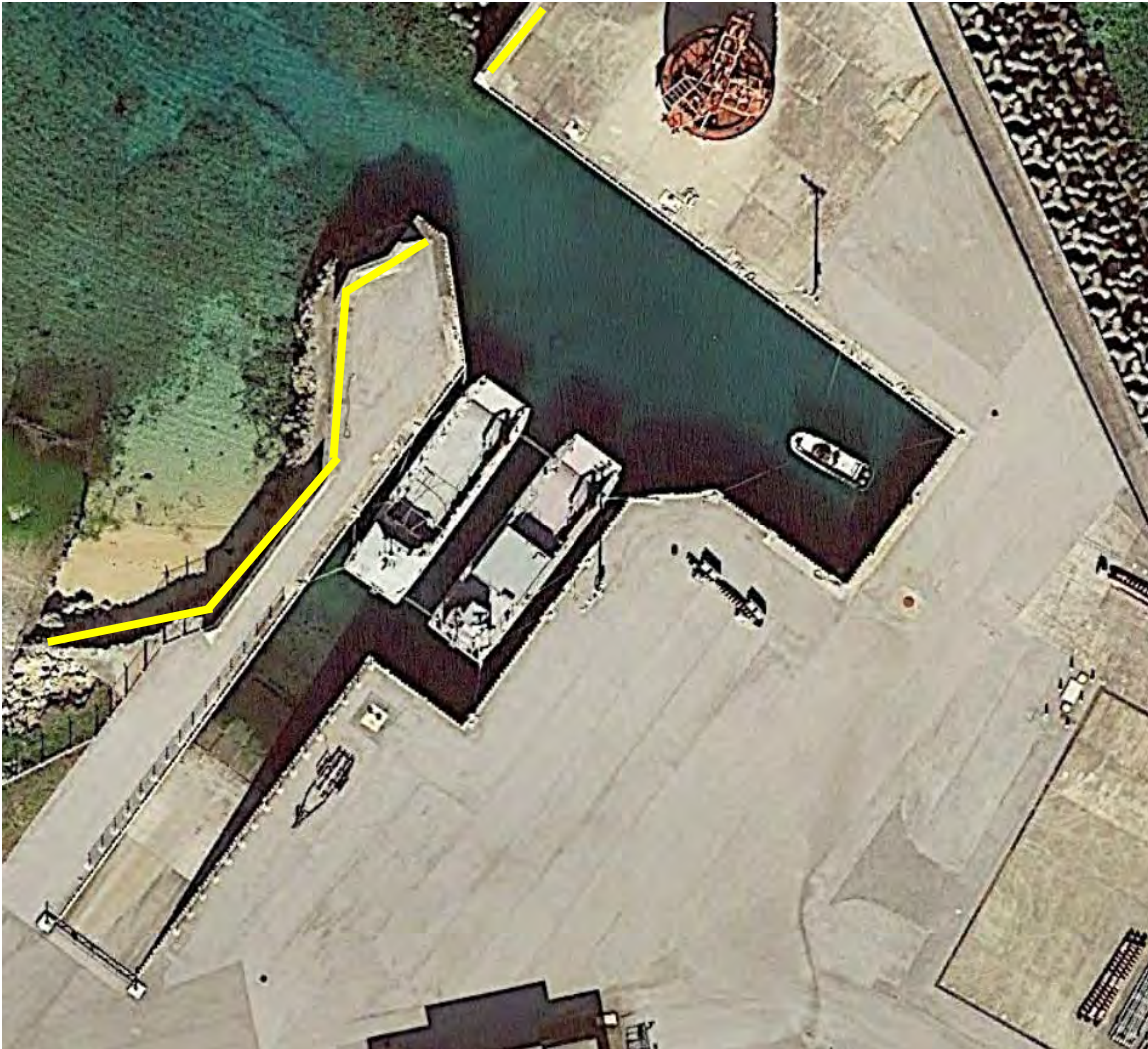
Figure 6-6. Aerial View of Tengan Small Craft Berth Seawall (Fac. Num: 312SW)
