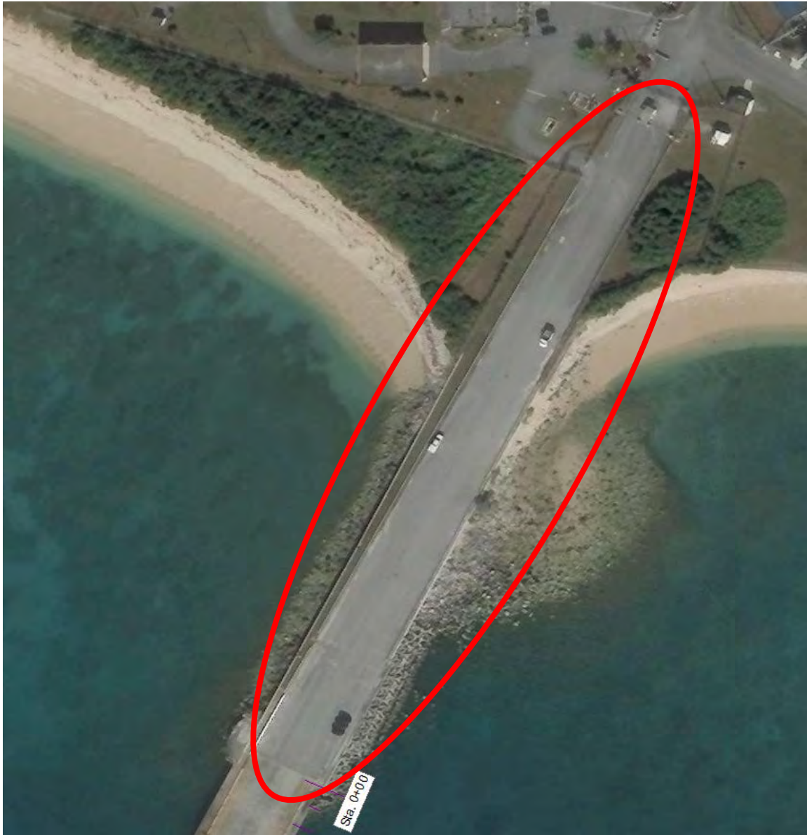
Figure 3-3. 800 LF Shore Attached Causeway
