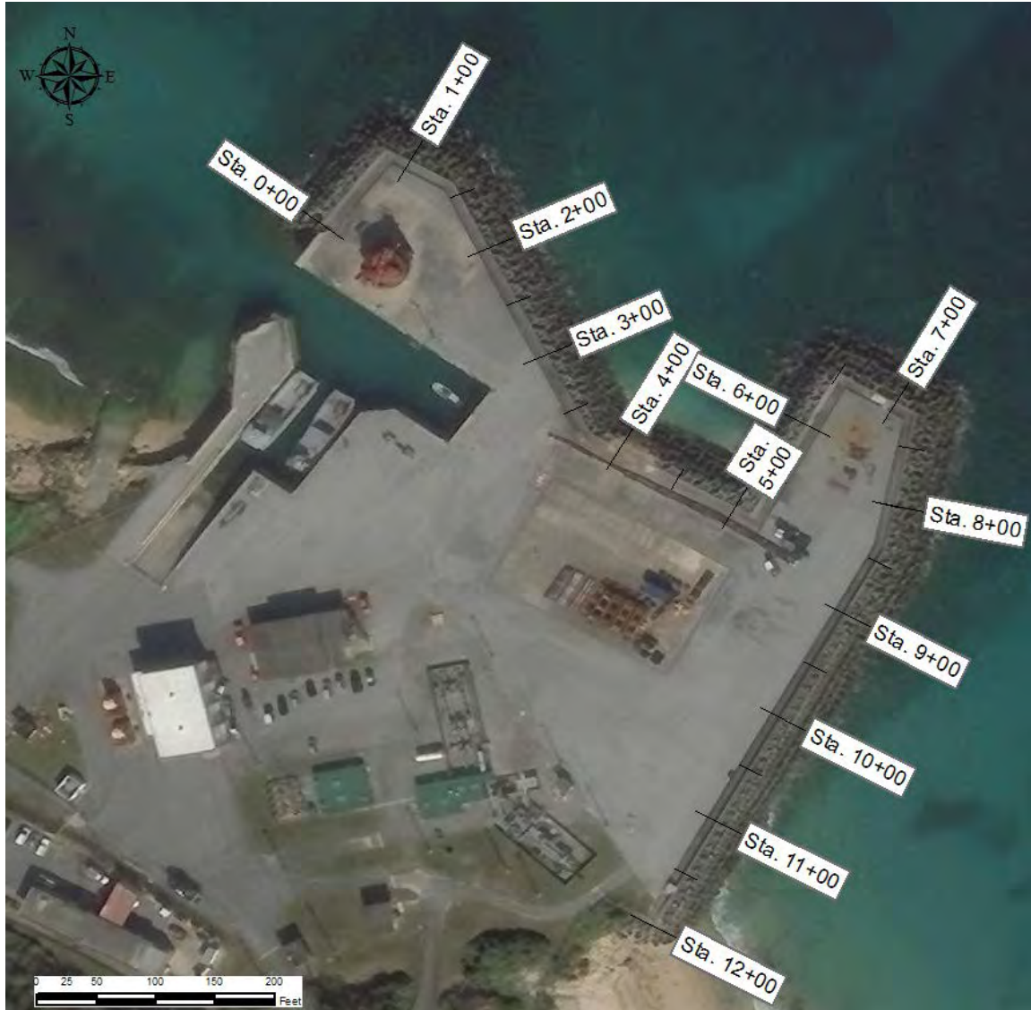
Figure 3-5: Tengan Small Craft Basin Seawall
