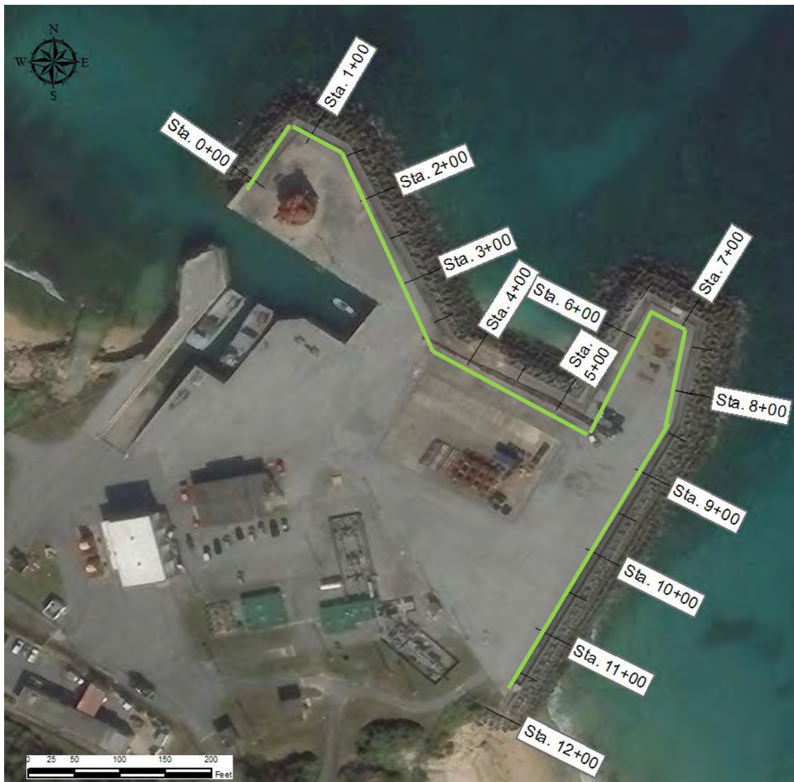
Figure 6-3. Aerial View of Tengan Small Craft Basin Seawall at CWTF#3 (15431)
