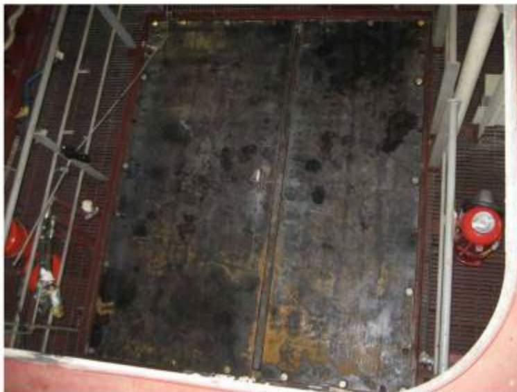
Figure, Z-drive Sea Well Covers Installed
