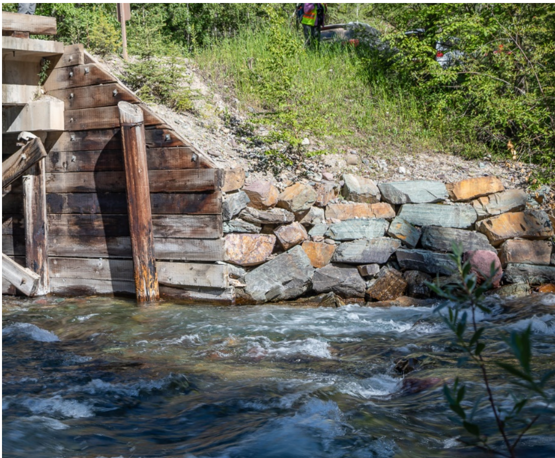
Stacked Boulder Revetment at Kintla Creek Bridge
