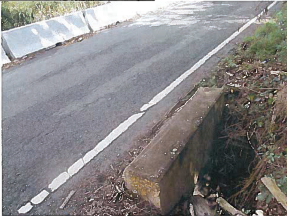
Figure 23: Photo 4 Culvert on the Southeast Side of the Section.
