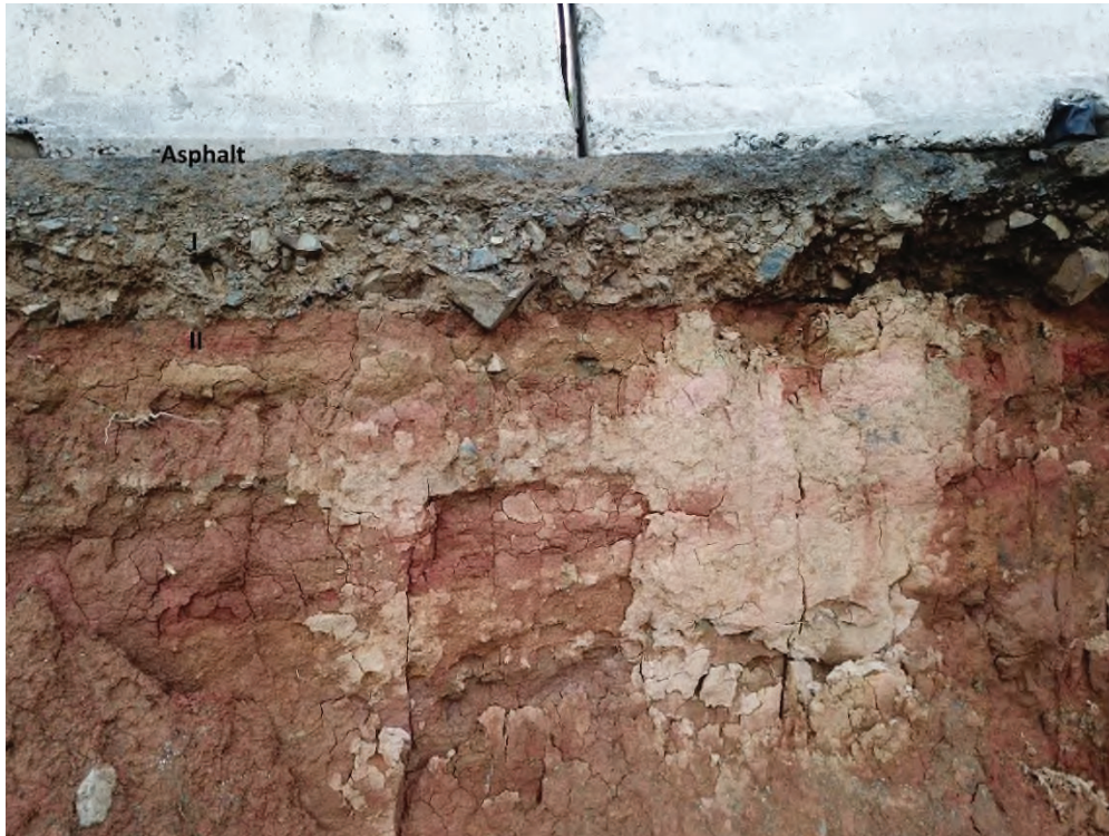
Figure 36: View of the Gap at km 13.0 Below the Asphalt It's the Brownish Layer Followed by the Reddish Clay
