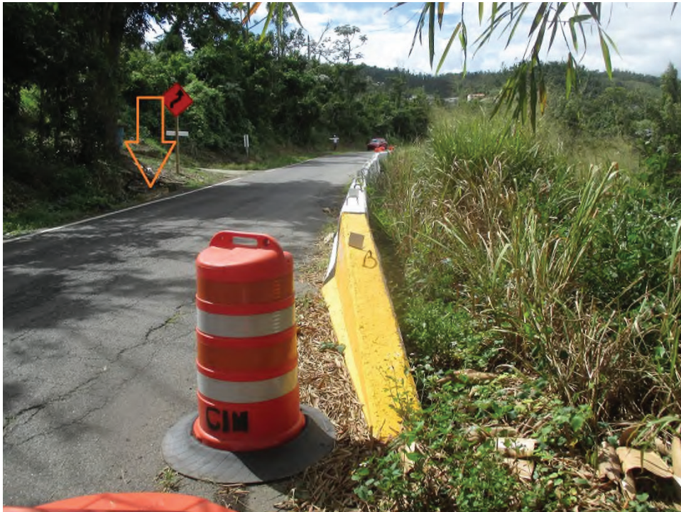
Figure 24: Photo 5 View Towards the Southwest of the Project. The Arrow Indicates the Place of the Storm Drain.
