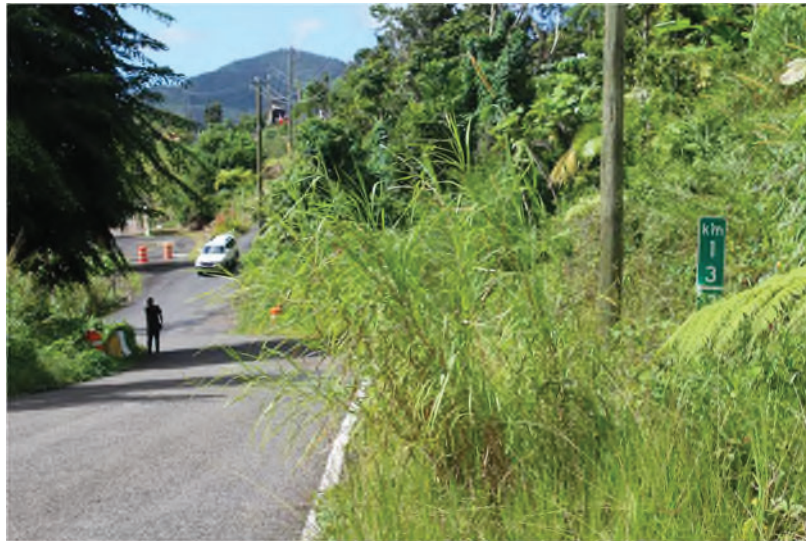
Figure 29: View of the Landslide from the 13.3 Mark.
