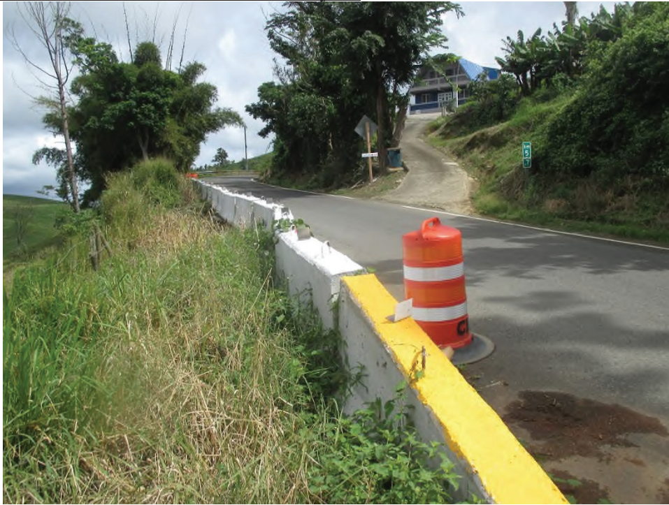
Figure 21: Photo 2 Concrete Barriers of Protection in the Project.
