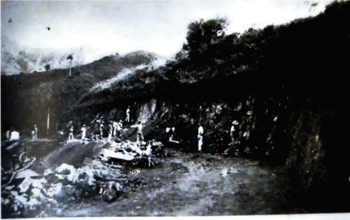
Figure 21: Photo of the Construction of the Road from Guayama to Carite, (Source: ROP VI:20 October 1929 :280)
