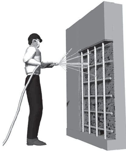
Fig. 3—Presaturate prepared surface with water.
