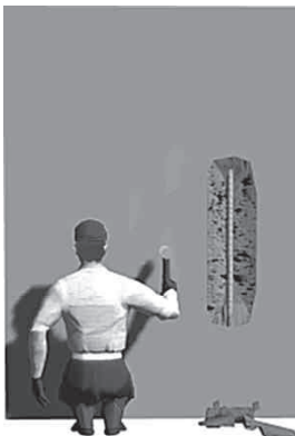
Sounding of concrete to locate areas of delamination.
