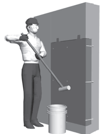
Fig. 4—Material placement: vertical application.
