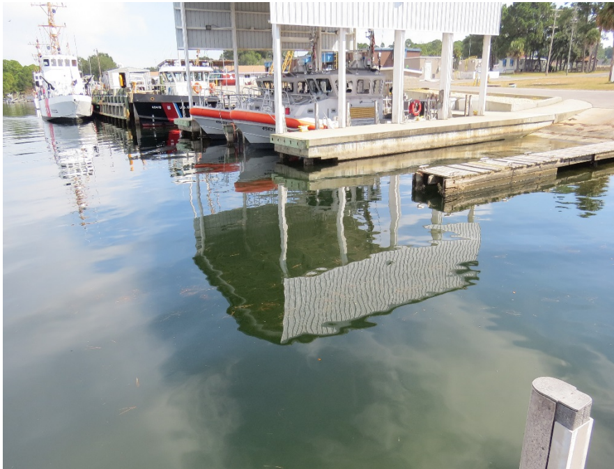
Photo 2: East side of project site, contains bulkheads and majority of structures.
