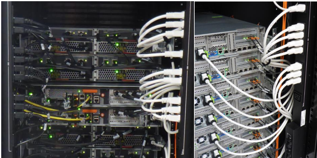
Figure 15: Example of Best-Practice Differentiated Power Cord Coloration Implementation
