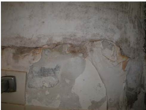
Deteriorated Finishes in bathrooms Dorms 902 and 903
