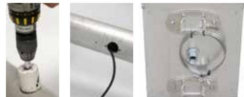
Excess cable can be left in the pole. If you'd rather trim cables, make note of their labels. Strip several inches off of the outer sheath of any cable that you've trimmed to length. Except for the solar panel wires, which already have ring terminals attached, strip each individual wire's insulation to expose about  $\frac{3}{8}$ " of bare wire. Slide a spade terminal fully over the exposed wire, then firmly crimp the terminal to the exposed wire.
