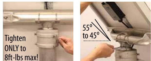
**Pole-side Mounted Solar Panel:** Band or bolt the bracket to the south side of the pole so it will receive the maximum solar input from the sun\*. Loosen the bolts that secure the pivoting arm to the pole bracket; then adjust the tilt of the solar panel pivoting arm to an angle of  $45^\circ$  above horizontal in southern latitudes, or a steeper  $55^\circ$  in northern latitudes. Tighten the bolts and nuts that secure the pivoting arm to the pole bracket.
