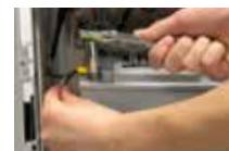
4. AFTER attaching Battery, attach Solar Panel leads:
