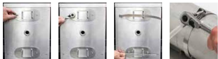
**Square Post/Flat Surface Mounts:** Feed a carriage bolt through each bracket. Place a bracket onto each set of studs. Place a washer, lock washer and nut onto each stud, then use a wrench to tighten the nuts. Feed the cables (fished out of the pole) in through the back of the control cabinet port. Feed the carriage bolts through post. Add a washer, lock washer and nut to each bolt and tighten with wrench.
