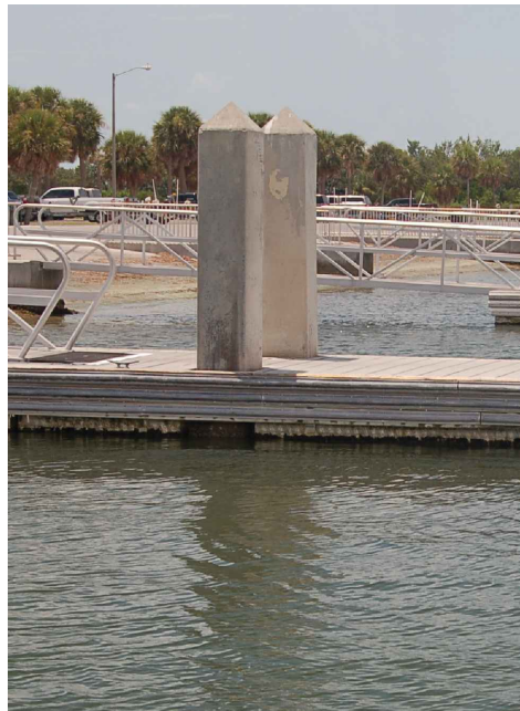
Concrete Piling
