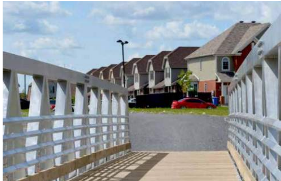
17 Wood and Aluminum Pedestrian Bridge
