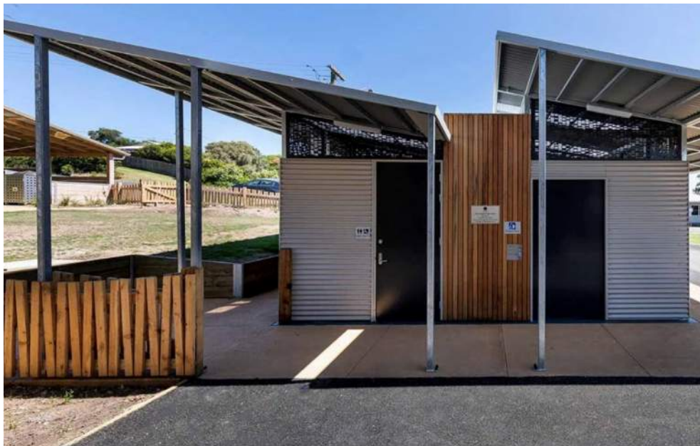
3 Wood and Metal Restroom with covered exterior
