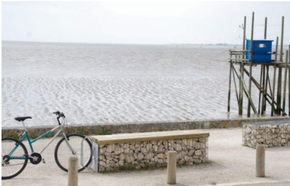
Bench – gabion base with bike rack
