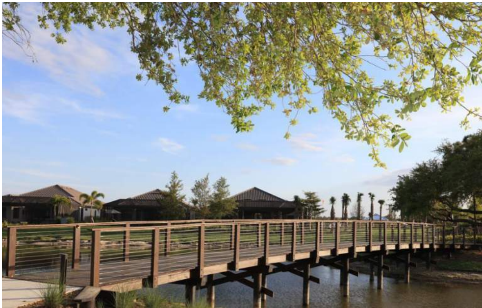
17 Wood Pedestrian Bridge
